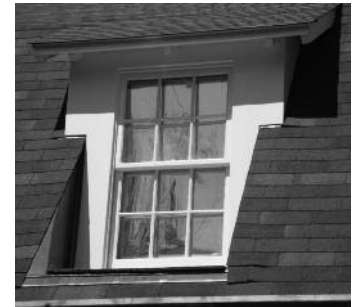
Window restoration, completed.
