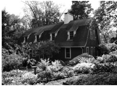
Before: Stepping Stones, looking as lovely as ever, but with triple-track storm windows, historically inaccurate shingles (which were badly weathered), leaking flashing, and aluminum gutters and leaders.
